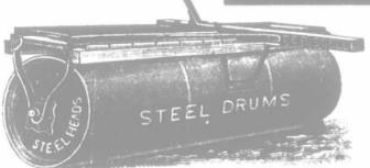
It rides easy. The position of seat prevents jars and jolts. Because of the large roller bearings, and because the axle revolves with drums, friction is reduced to the vanishing point. The "Bissell" is the lightest draft, as well as the easiest riding and smoothest soil packer on the market. For further particulars ask Dept. W. for catalogue, or see your local dealer.
