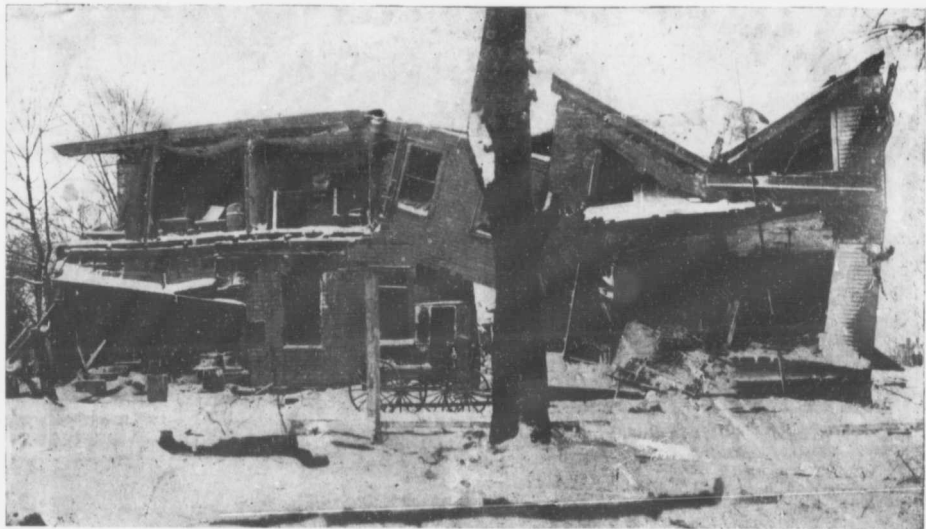
WRECKAGE OF SHOP AND HOUSE IN THE DEVASTATED AREA. Furniture can be seen among ruins.
