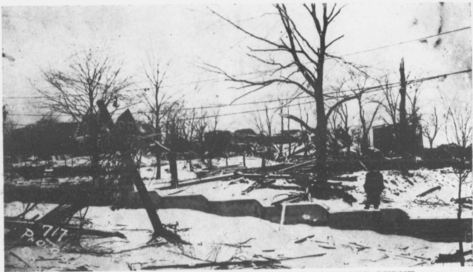
KAYE ST. METHODIST CHURCH WAS BLOWN DOWN AND BURNT. Note foundation in the foreground.
