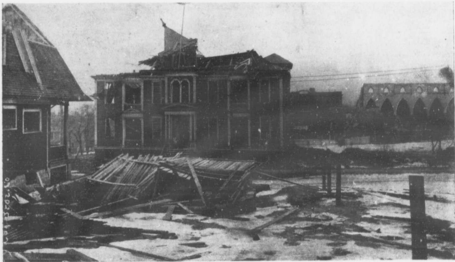
Although many Blocks away St. Joseph's School was badly shattered. Part of St. Joseph's Church is also shown at extreme right.
