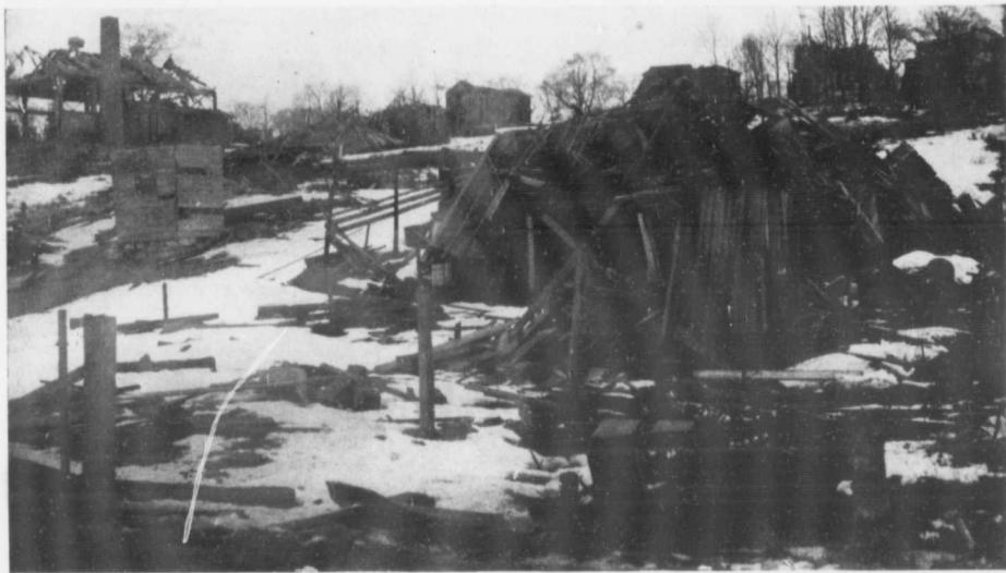
WRECKED HOUSES IN DARTMOUTH, Opposite scene of explosion.
