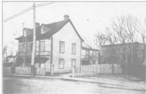
GEORGES ROY 60 Fraser General Contractor Entrepreneur Général
