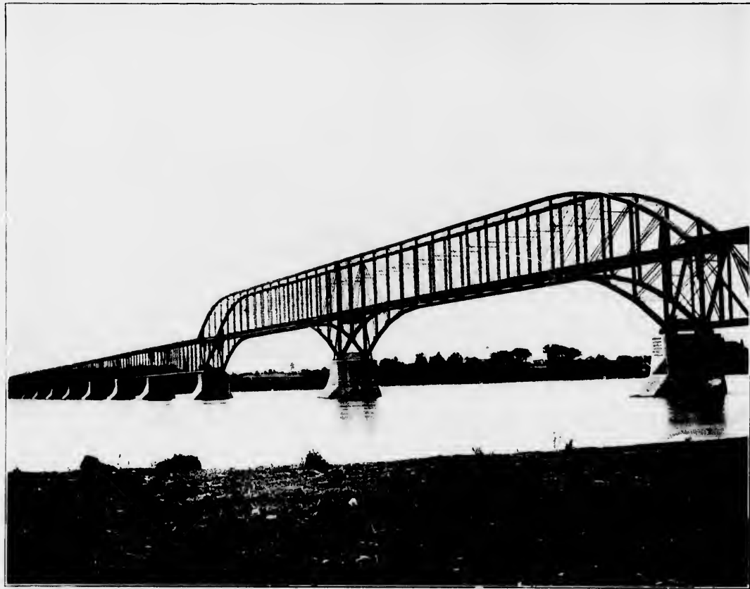
THE CANADIAN PACIFIC RAILWAY BRIDGE.
