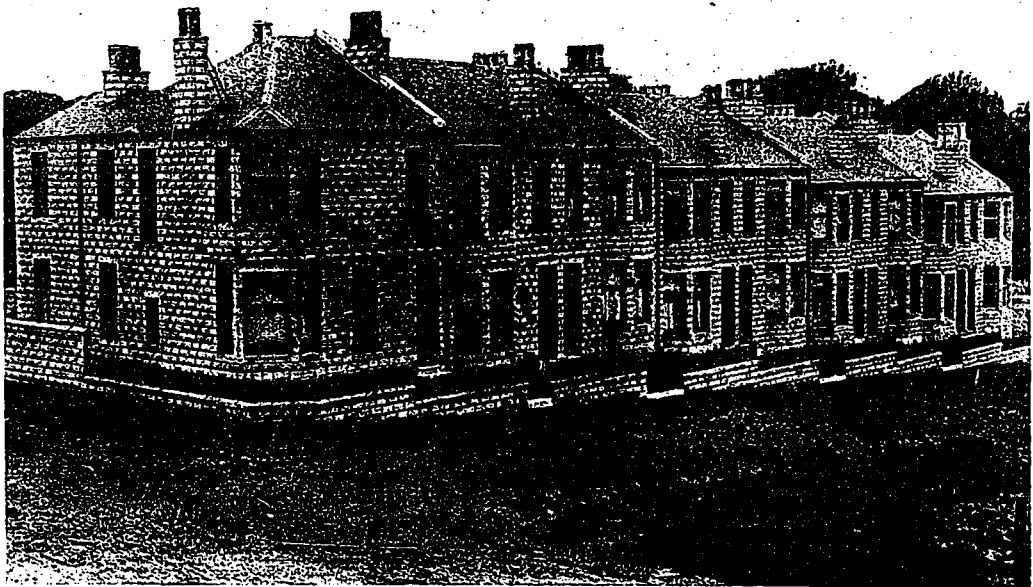
Terrace of concrete block houses at Burnside (near Glasgow), Scotland, providing accommodation for nine families. This illustration shows how well adapted this material is to meet the needs of economical and well constructed dwellings of the attached type.
