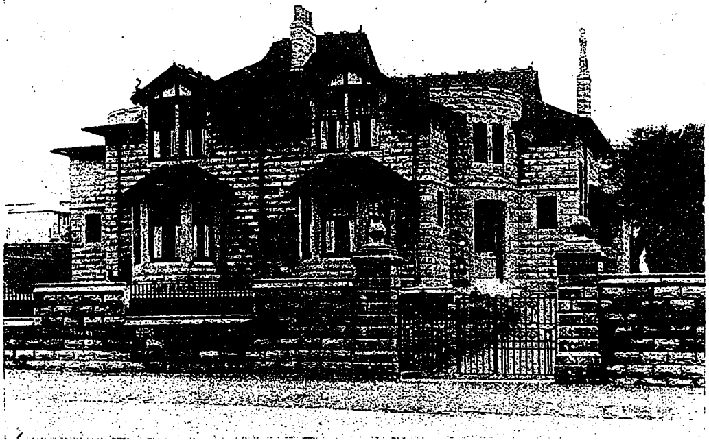
This house shows the introductory use of concrete blocks in Scotland. It is a two-family dwelling located on the main Glasgow Road, Paisley, and was the first concrete block house built at that place. Note how carefully the architectural and constructive detail has been considered and the thorough manner in which the work has been executed.
