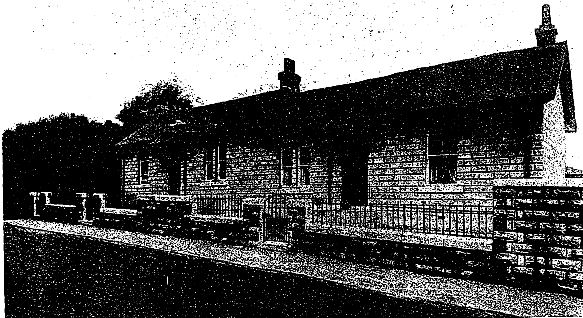
Two family cottage at Dumbarton, Scotland. A simply and pleasingly designed small double dwelling, executed in concrete block, the front of the building being of panel blocks, while the remaining portion of the walls is carried out in blocks of the rock-faced type.
