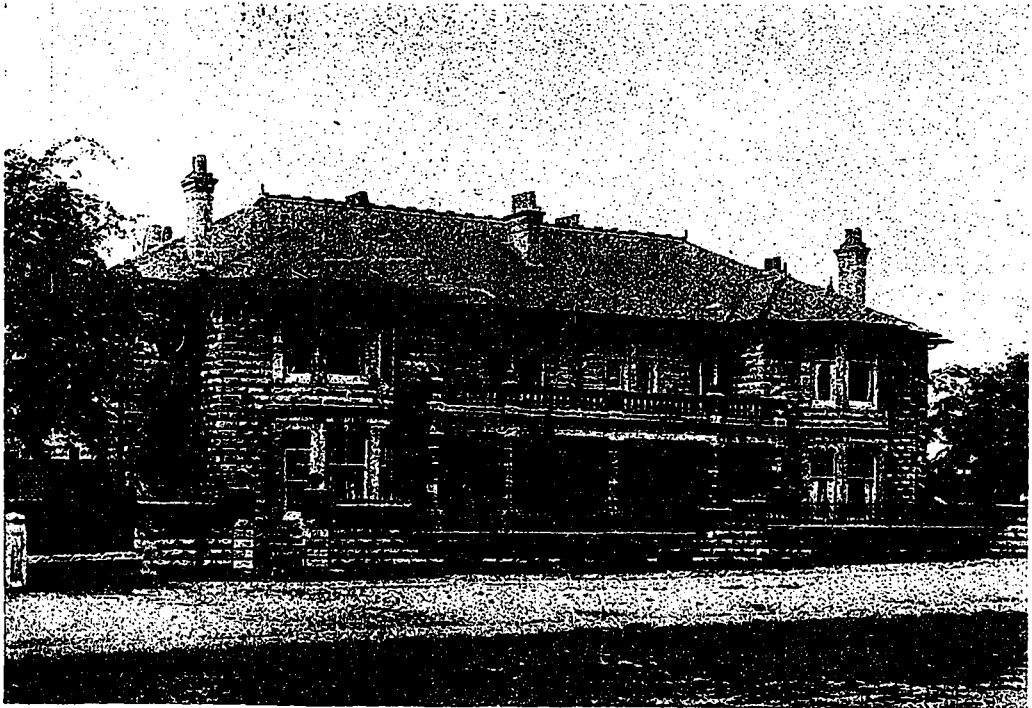
Four family concrete block house, Paisley, Scotland. Note how monotony of rock face is relieved by introduction of panel blocks and broken ashlar effects.
