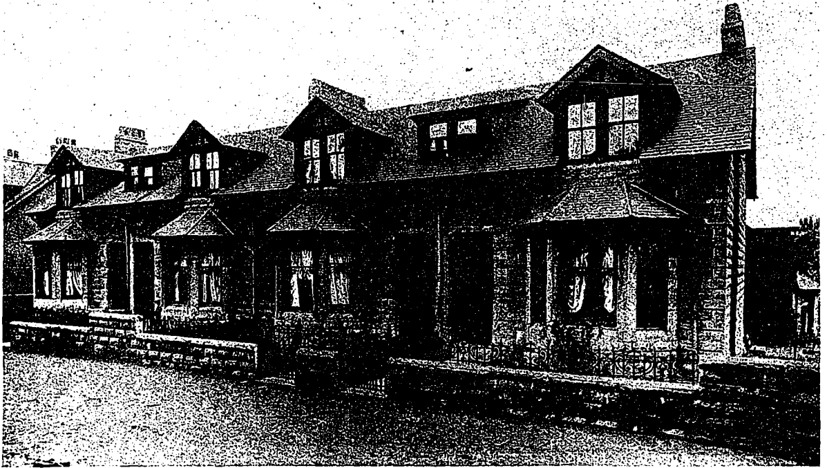
Four family cottage, built of concrete blocks, at Paisley, Scotland, where this form of construction is coming much into evidence.
