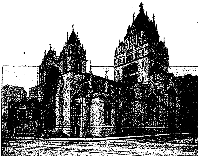
The Broadway Tabernacle (Congregational), Broadway and Fifty-sixth street, New York, designed by J. Stewart Barney. While thoroughly ecclesiastical in character, this church is remarkable as combining, on a limited site, a large auditorium and a twelve-story office building for parish work.
