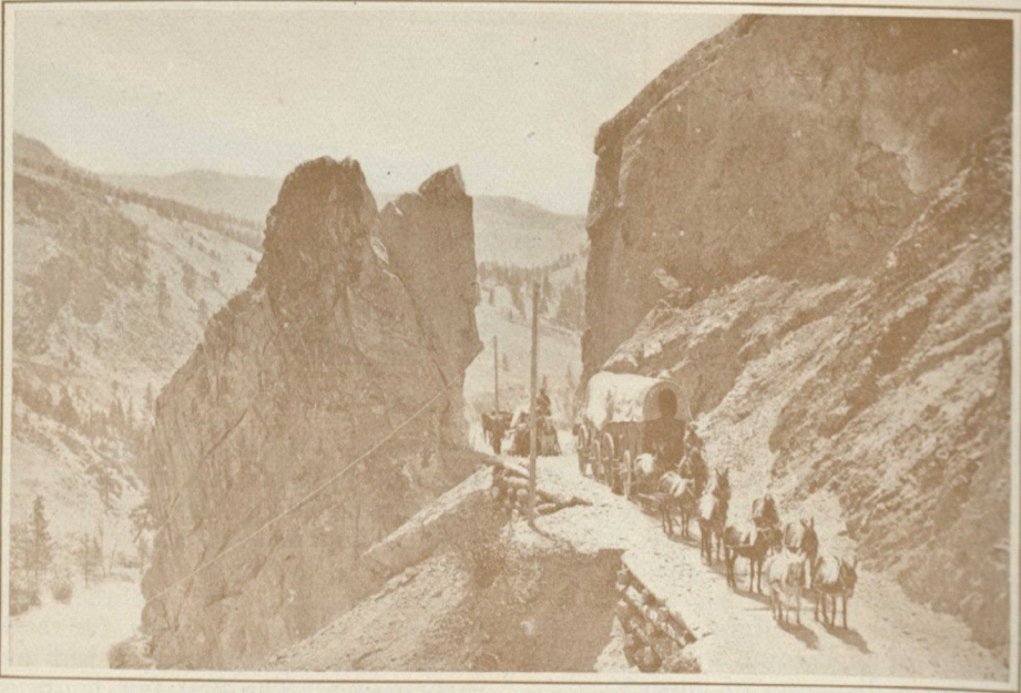
A FIVE-SPAN HAUL UP GRADE
