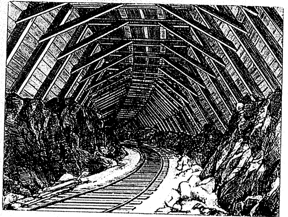
INSIDE OF SNOW-SHED AT METAPEDIA.
