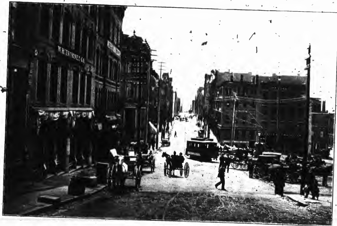
PRINCE WILLIAM STREET, LOOKING SOUTH.
