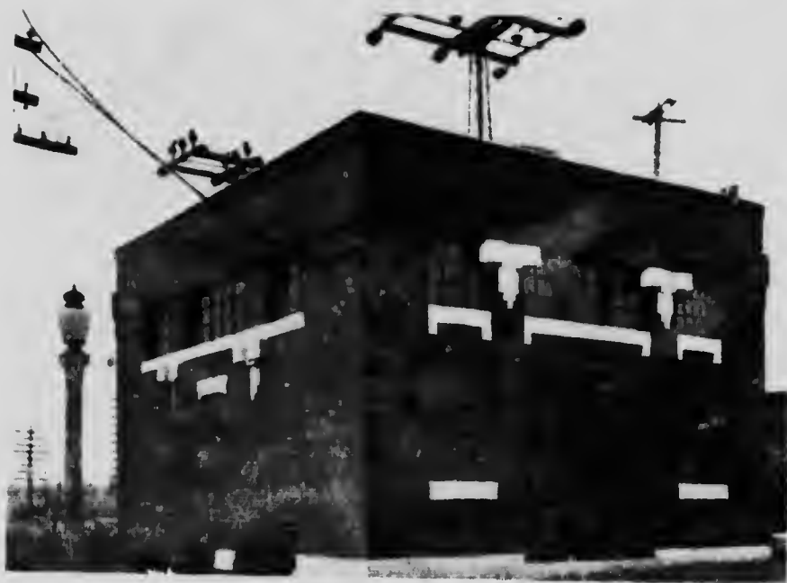
Fig. 1,945. An Automatic Substation on the Great Lakes.
