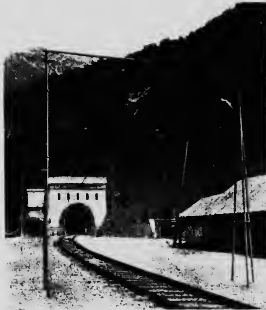
FIG. 105. Three-phase Overhead Construction in the Alps (the Simplon Tunnel).
