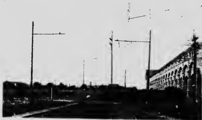
Fig. 1,693.—Curves and Junctions in Catenary (Bracket) Construction.
