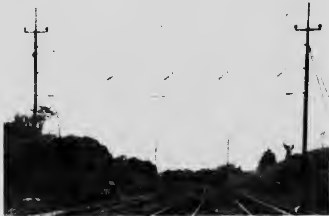
Fig. 1,691.—Single Catenary (Span-wire) Construction on a Sharp Curve
