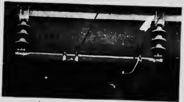
Fig. 175.—Catenary passing under a Bridge.
