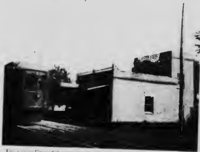
Fig. 1,941.—Union Sub-station on the Elgin and Belvedere System, a Pioneer Automatic Sub-station (1914).
