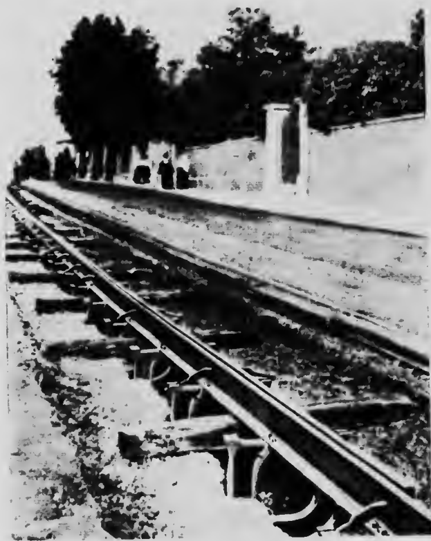
Fig. 1,534.—Slot Rails and Yokes in Position.
