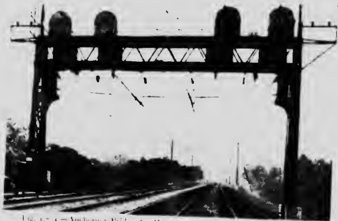
Fig. 174.—Anchoring Bridge for Catenary Suspension on the Pennsylvania Railway (1910)
