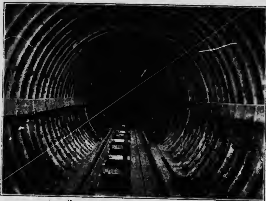
Fig. 1,651.—The Interior of a London Tube Railway.
