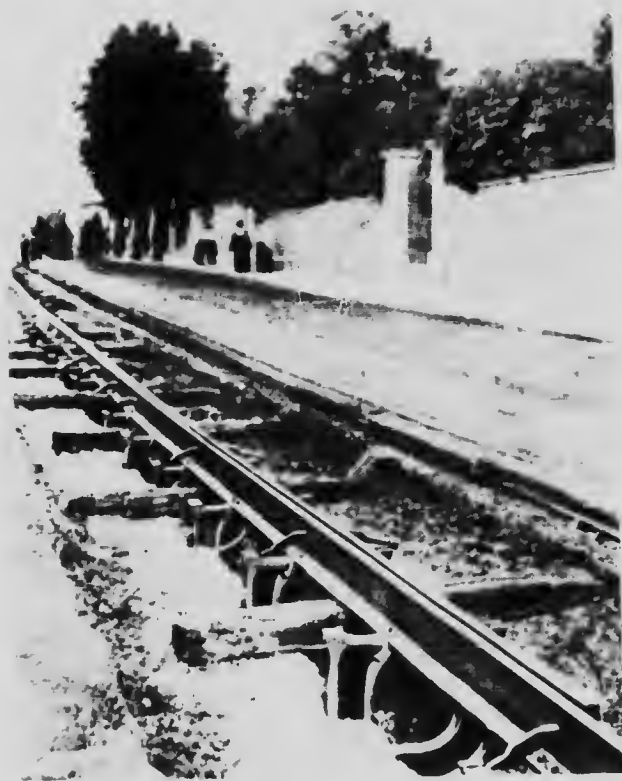
FIG. 1,534. Slot Rails and Yokes in Position.
