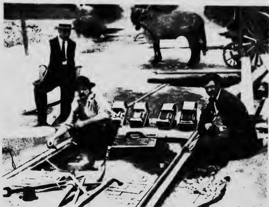
FIG. 1759.—Rail Welding, "Insert" Thermit Method
