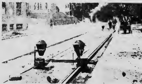
Fig. 1,761.—Preheating the Mould, Before Welding
