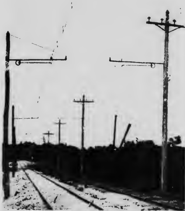
FIG. 1-85.—Typical American Single Catenary Suspension (cont'd).
