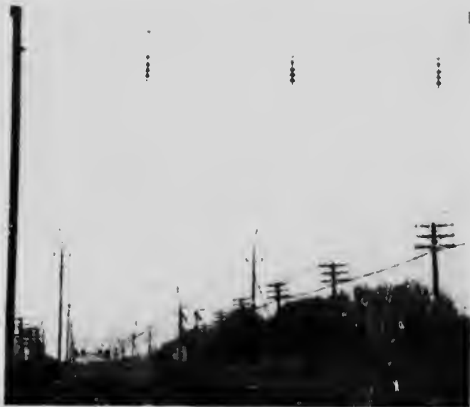
Fig. 1660. Single Catenary with Span wire Suspension.
