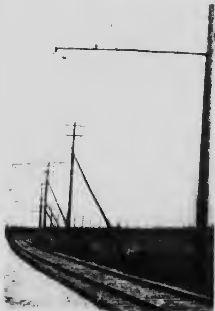
Fig. 1661. Single Catenary Construction on a Curve.
