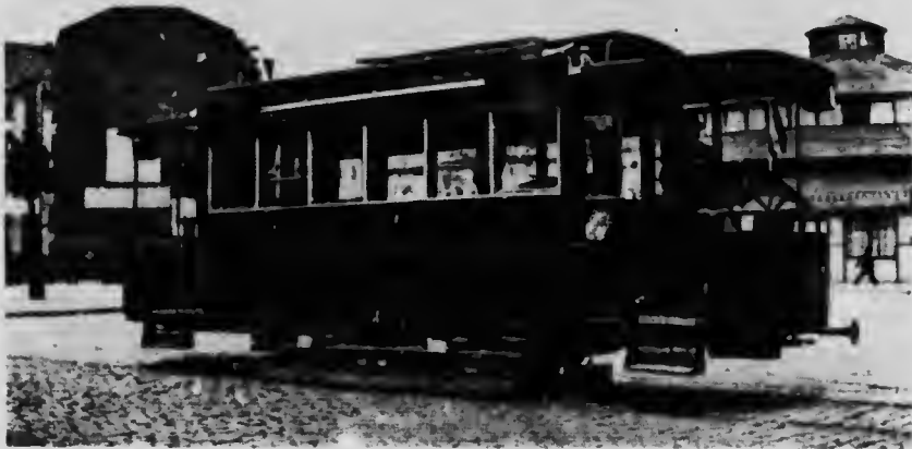
Fig. 1,588.—Tramcar Propelled by a Secondary Battery.
