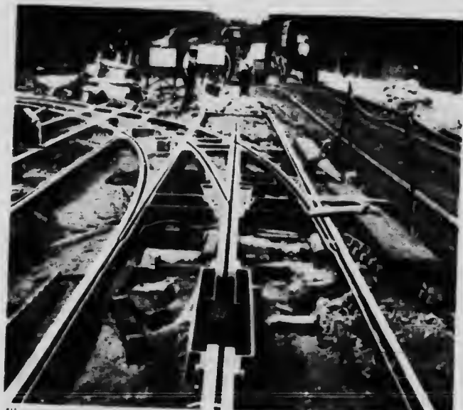
Fig. 1,544.—A Portion of an Unfinished L.C.C. Track before the Paving is Laid.
