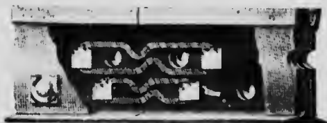
Fig. 1,746.—Double Bonds Protected by Hat Fish-plate.
