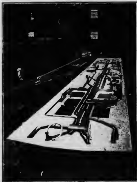
Fig. 1, 87. Wiring underneath the Floor of a Motor Coach for Single-phase Working.
