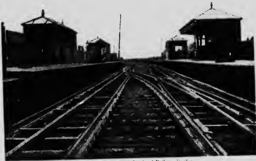
Fig. 1,643.—The Liverpool Overhead Railway in 1893.
