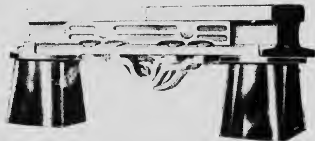
FIG. 1,753. Bonding of Conductor Rail in Hudson River Tunnel.
