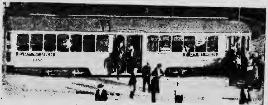
Fig. 1,830.—Typical Modern American Trolley.
