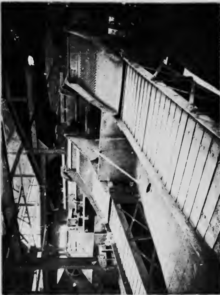
Front end of belts showing arrangements for elevating and delivery, Clock Face colliery, England
