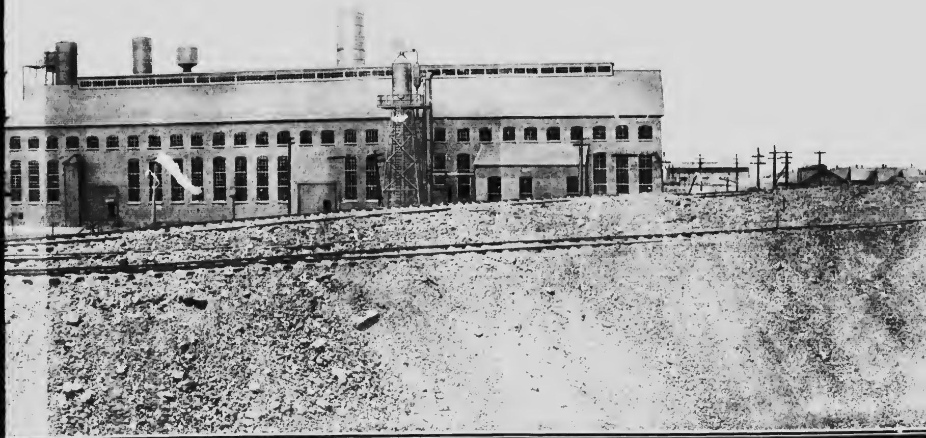
16. S., showing bankhead, main shaft, hoisting engine house, power house, and part of winter's accumulation of banked coal, approximating 300,000 tons.
