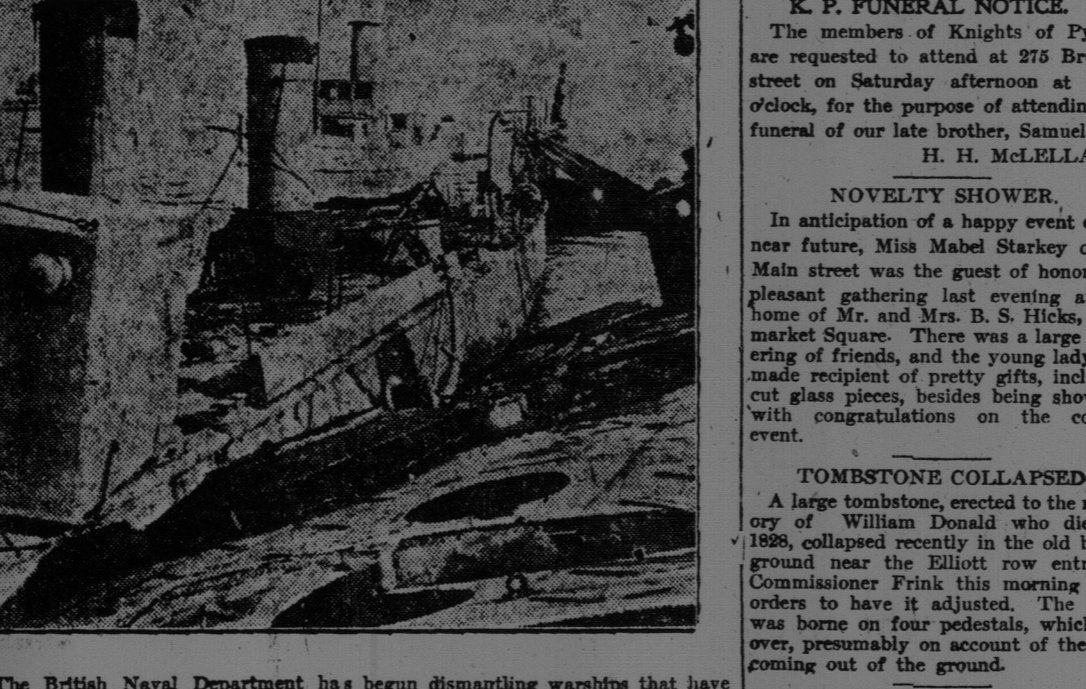
The British Naval Department has begun dismantling warships that have become out of date. Here are two destroyers being broken up.
