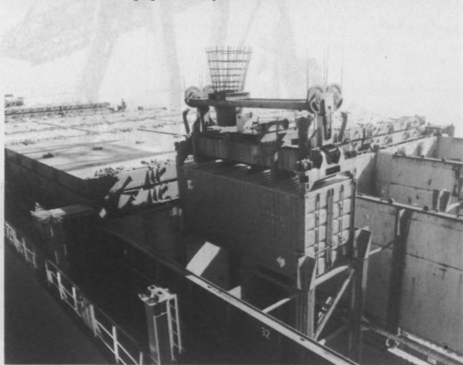
*Container crane loading container into cellular containership.*
