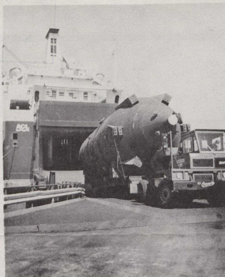
A 50-ton, stainless-steel-lined Batch Digester is loaded at the Port of Montreal. The Digester, manufactured by Horton/CBI of Fort Erie, Ontario is being exported by H.A. Simons (Overseas) Ltd. to a sulphite pulp mill in Ruzemberok, Czechoslovakia. The $300-million project was financed by loans of $218 million by EDC, and $80 million by a consortium of Canadian banks.
