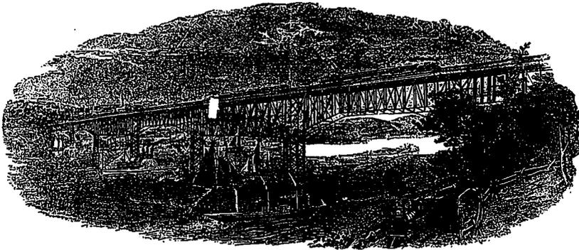
world. It will consist of five spans over the river channel, three of them cantilevers 550 feet each, and two truss spans of 525 feet each. The material is steel, and will be supported on tall steel towers resting upon stone piers 252 1/2 feet on top.
