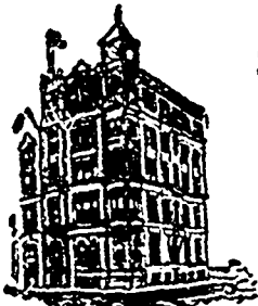
HEAD OFFICE BUILDING, MONTREAL.
