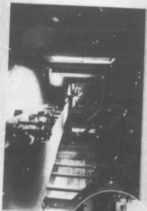
HOW GRAIN IS CONVEYED BY BELTS.
