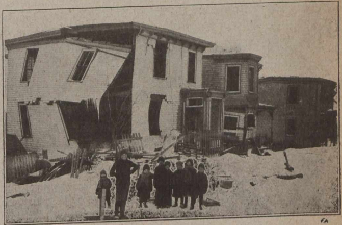
Typical View of Streets Bordering the Devastated Area
