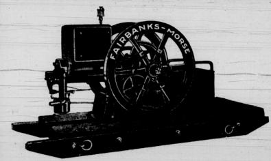
This type has no equal for outdoor service in all weathers for crushing, sawing, etc. It is hopper cooled and mounted on substantial iron shod skids.
