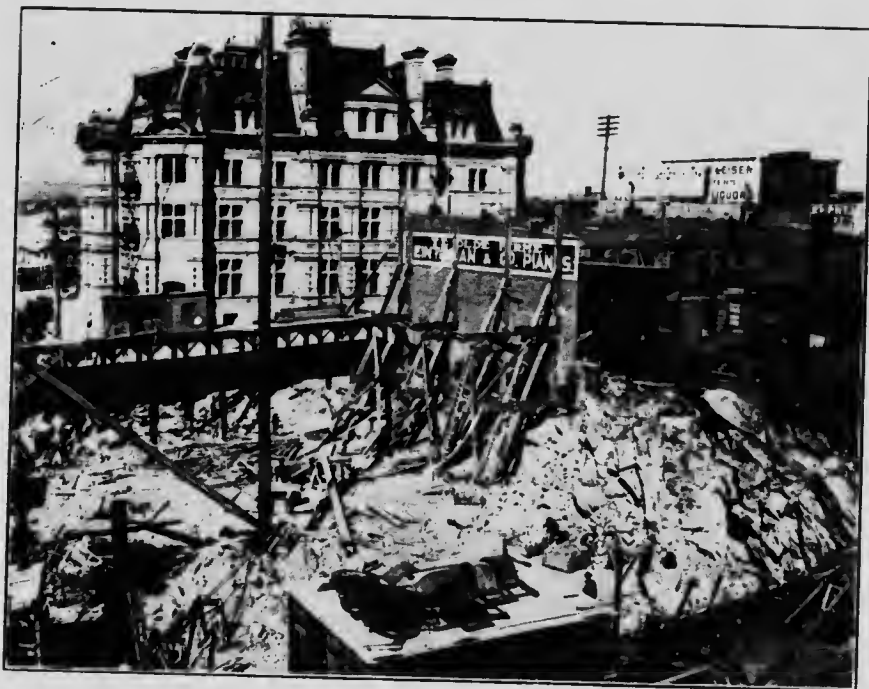
Rock Cut for Foundation of 8-story Block opposite Custom House
