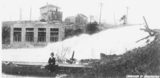
USINE HYDROELECTRIQUE DE LA GANANOQUE ELECTRIC LIGHT AND WATER SUPPLY CO., A KINGSTON MILLS, CO. DE FRONTENAC, ONT.
