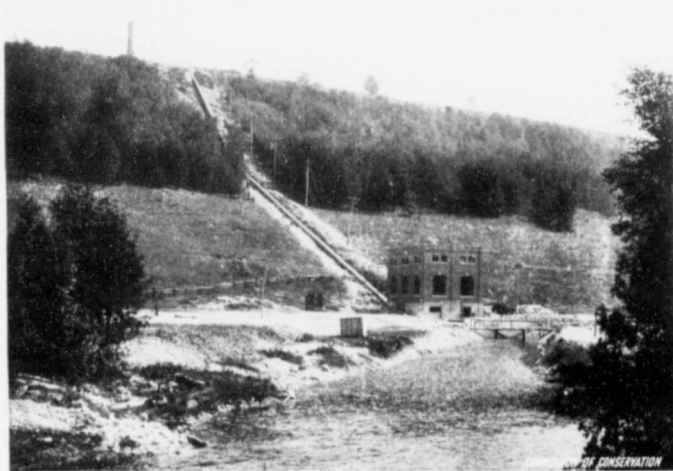
USINE HYDROELECTRIQUE DE LA ONTARIO HYDRO-ELECTRIC POWER COMMISSION, AUX CHUTES EUGENIA, CO. DE GREY, ONT.
