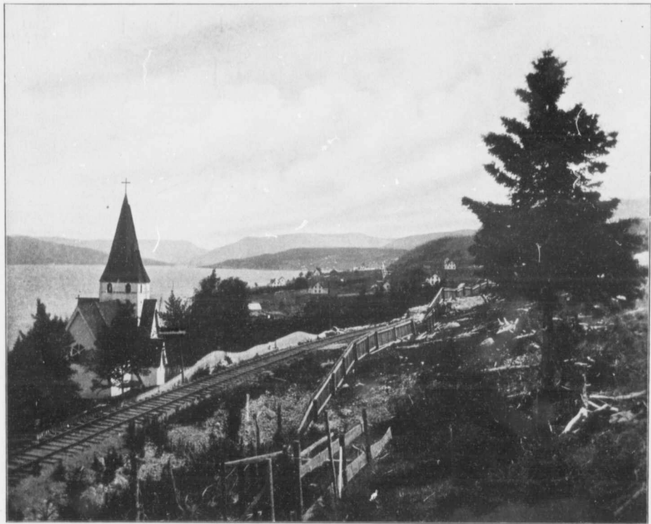
63. RAILWAY PASSING THROUGH BIRCHY COVE—BAY OF ISLANDS. Looking towards the entrance to the Humber River.
