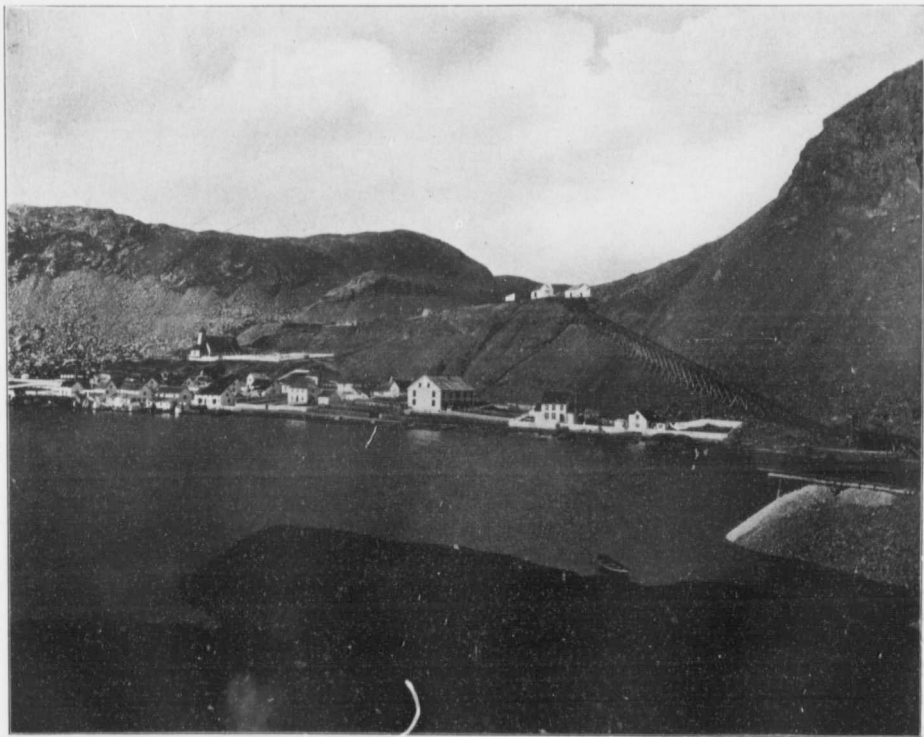
115. TILT COVE COPPER MINE, NOTRE DAME BAY.
