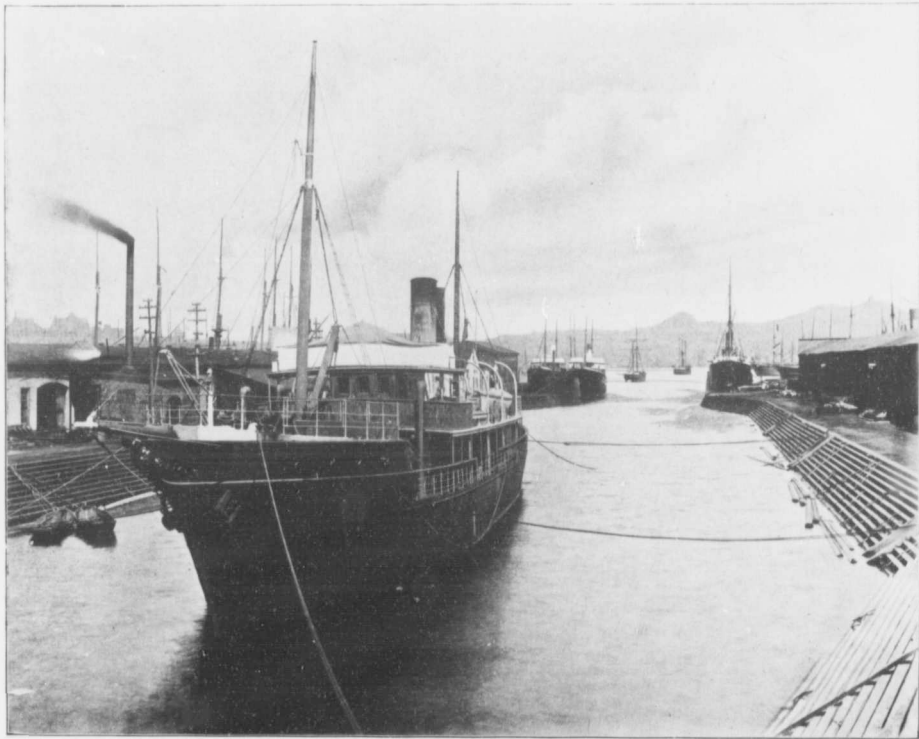
12. ST. JOHN'S DRY DOCK.
