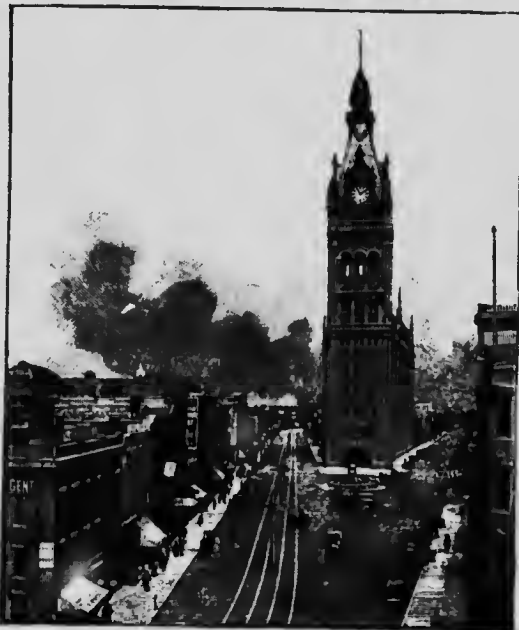
FIG. 73.—CITY HALL, MILWAUKEE.
