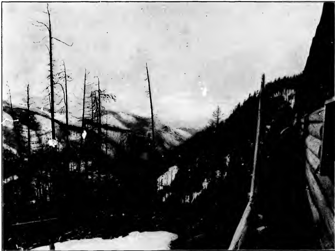
LOOKING DOWN SHEEP CREEK CANYON FROM MINE.
