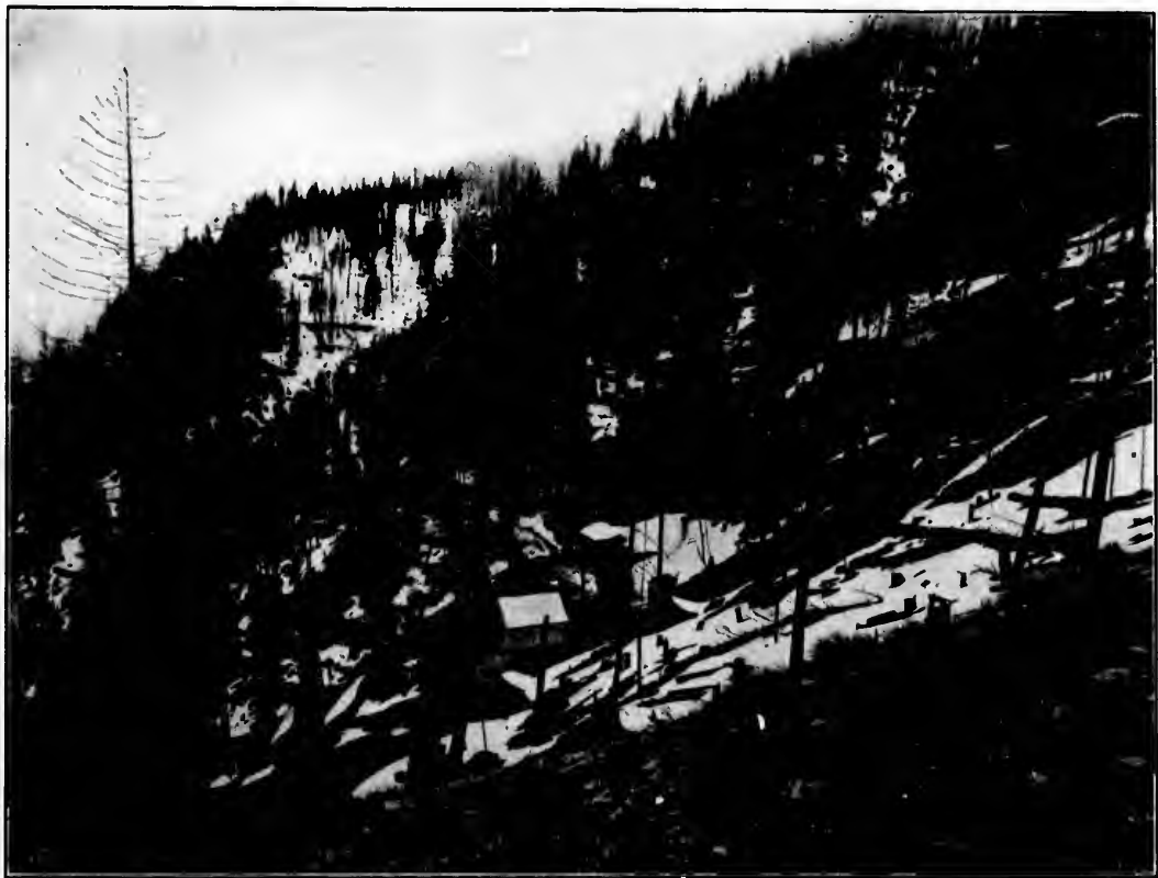
UPPER TERMINAL OF AERIAL TRAMWAY AT PORTAL OF NO. 5 TUNNEL TO 500 FT. LEVEL OF MINE, 2000 FT. ABOVE MILL.
