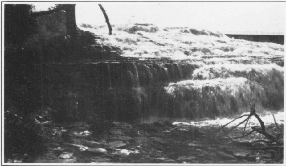
View of Healey Falls, which supplies part of the power for the Commission's Central Ontario System.
