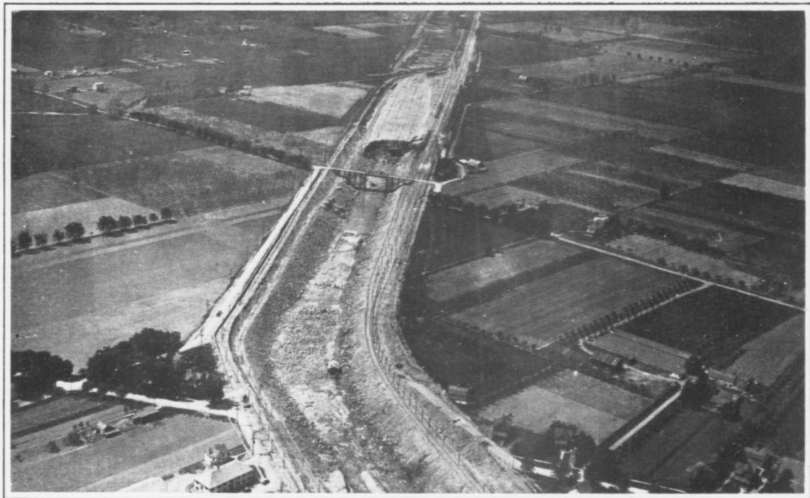
Aeroplane view of the Queenston-Chippawa Power Canal under construction.
