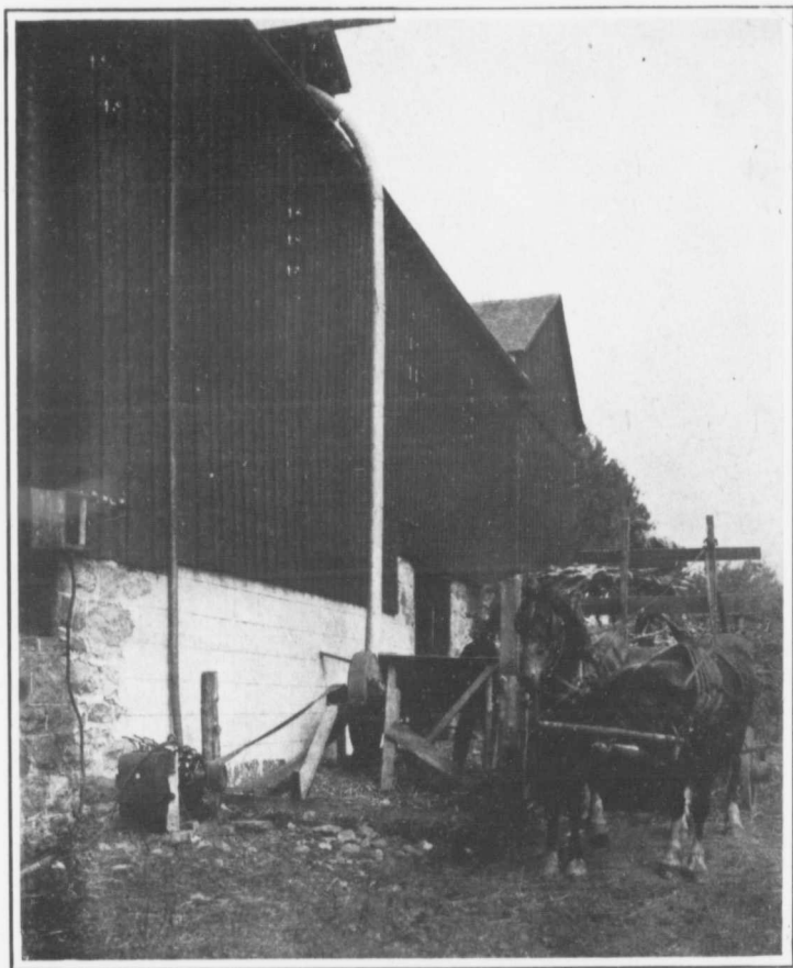
Silo-filling with Hydro Power.
