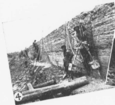
(1) Cableway Excavator in Welland River. (2) Cableway Excavator from East Bank of Welland River. (3) Site of the World's Largest Power House. (4) Drilling wall of Forebay. (5) Dredge loading scow opposite Hog Island, at the mouth of the Welland River.
