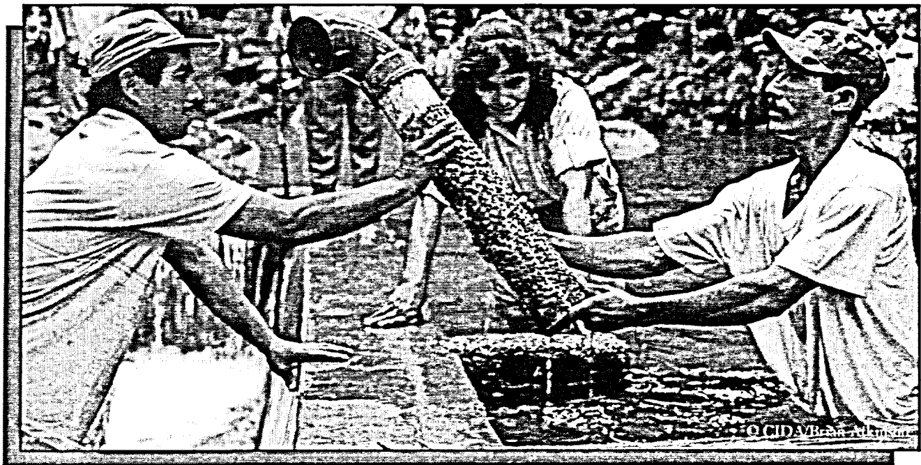
Workers clean the filters of a dam in Palos de Agua, Honduras, as part of the Sustainable Water and Sanitation Project.
