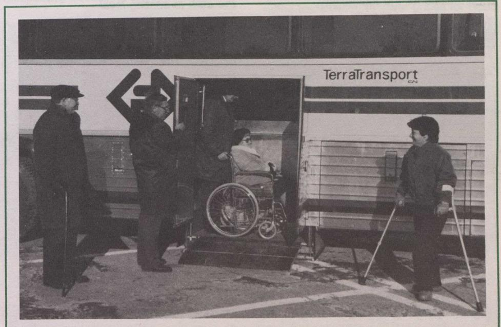
Inside elevator on intercity bus allows easy access for disabled passengers.
