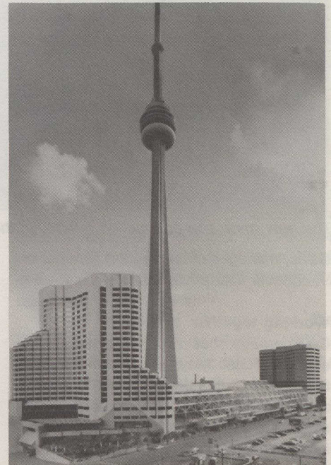
The $90-million convention centre complex in Toronto, with the impressive CN Tower in the background. The centre, which hosted its first convention this summer, can accommodate groups of up to 12 000.
