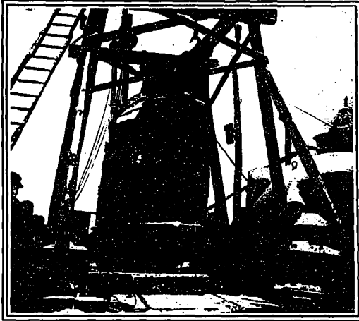
METHOD OF UNLOADING 55-TON TOP CASE OF THE WATER WHEEL.
