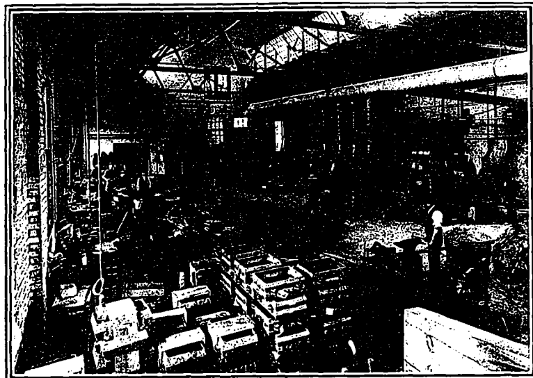
FOUNDRY 50 FT. X 100 FT. IT IS A BRICK AND STEEL STRUCTURE. THE FLOOR IS 4 IN. OF CONCRETE WITH 1 IN. OF SAND AND VITRIFIED BRICK ON EDGE.
