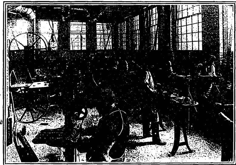
THE PATTERN ROOM ON THE SOUTH SIDE OF THE BUILDING, ADJOINING THE TOOL ROOM, IS ONE OF THE MOST IMPORTANT ADJUNCTS TO AN UP-TO-DATE BRASS PLANT.
