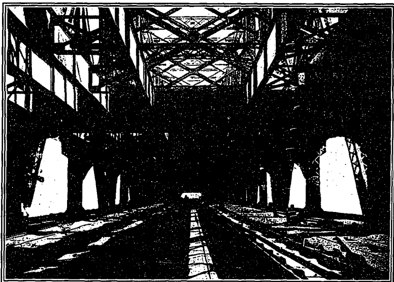
VIEW LOOKING THROUGH BLACKWELL'S ISLAND BRIDGE, NEW YORK, FROM THE LOWER DECK, SHOWING THE MASSIVE STRUTS AND BEAMS, ALSO THE HEAVILY INTER-LACED VERTICALS AND DIAGONALS.
