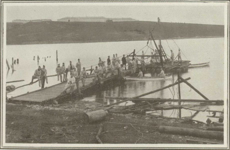
BRIDGE-BUILDING AT THE ROYAL MILITARY COLLEGE
