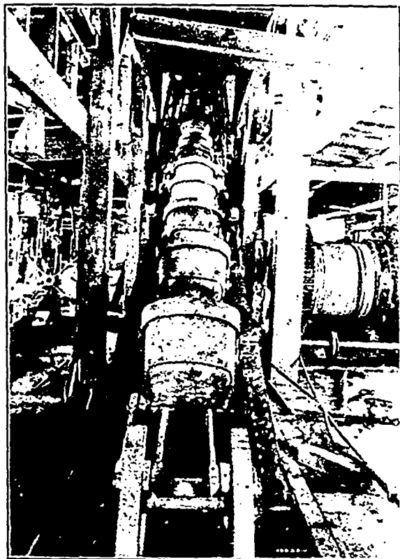
Dredge at Lillooet—72-ft. Steel Bucket Ladder. Buckets and Engines.
