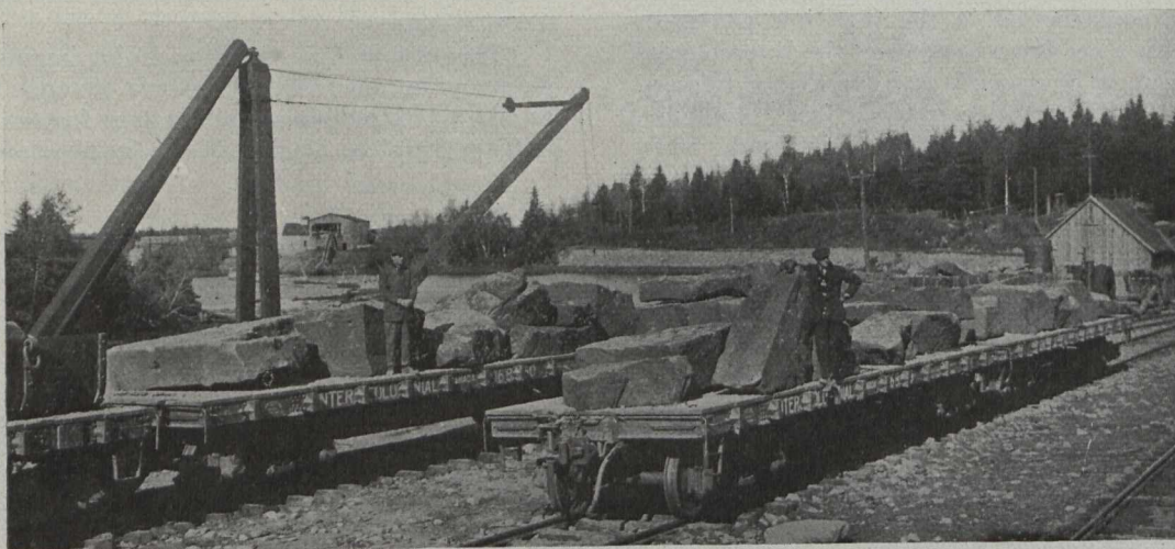
Rock Used in Facing Pier and Breakwater.
