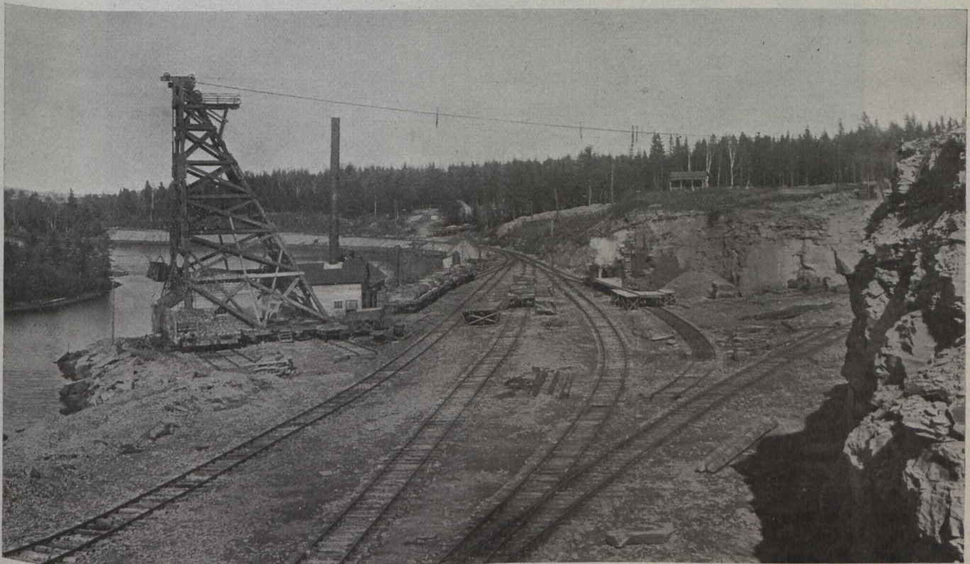
General View of Quarry Yard, Showing Track Layout, Cableway and Rock Formation.
