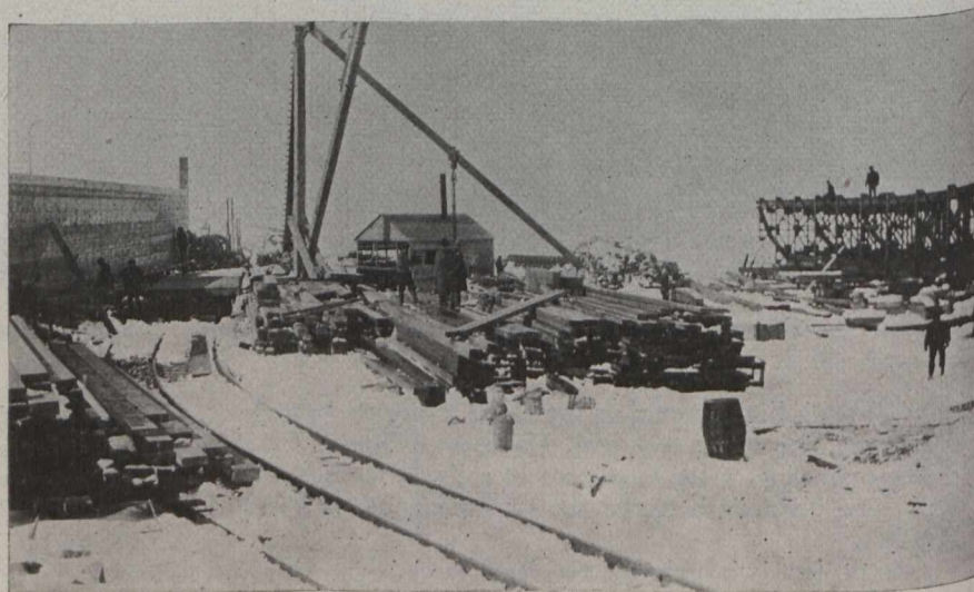
Dry Dock and Steel Deck Scow Under Construction at Point Du Chene.
