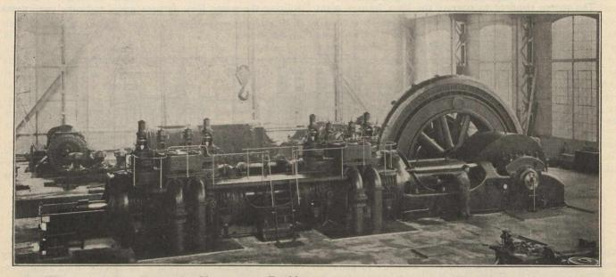
Showing One of Two Units, 1800 Horse-power Double-acting Nurnberg Engine at Gilsenkirchen, Operated by the Aktien-Gesellschaft Schalker Gruben-u. Hutten-Verein, and Installed by the Vereinigte Maschinenfabrik Augsburg und Maschinenbaugesellschaft Nurnberg, A.-G. Work, Nurnberg.
