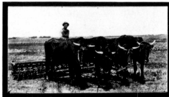
The packer should follow the breaking plow
