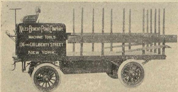
sectional trays which slide out at either side. The power is furnished by two motors of General Electric make, operating independently on rear wheels. Tires are 6-in. solid rubber. Forward springs are full elliptic, the rear one-half elliptic. A double brake operates on inside of gear wheels, being worked by foot pressure. The controller has four speeds ahead and two reverse, maximum speed of truck
