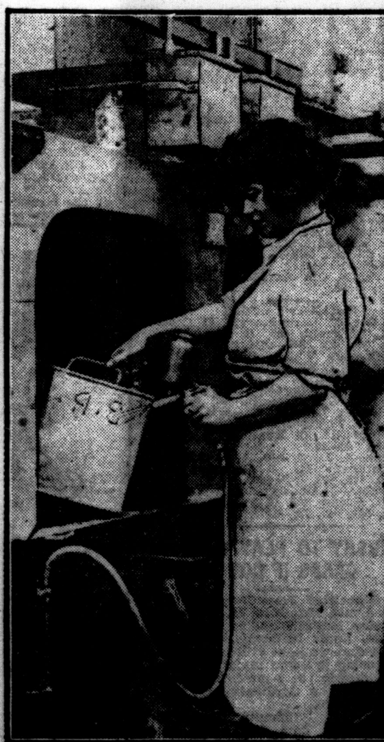
In canning gasoline for motorists, all empty cans are inspected with electric torches for dirt and dust. They are then tested by compressed air for leaks. Girls in London are shown painting the cans by air brush
