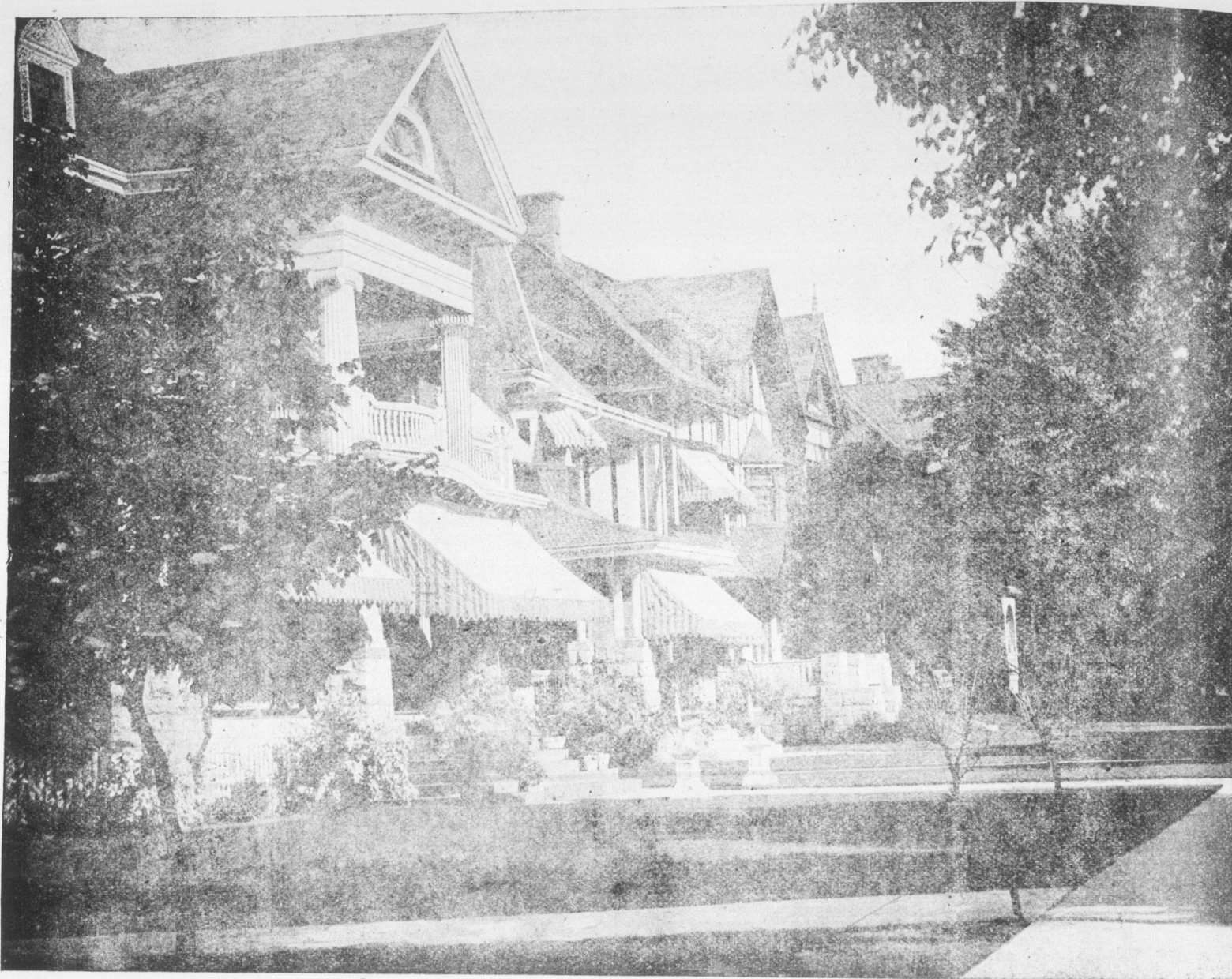
RESIDENTIAL STREET OVERLOOKING VICTORIA PARK.
