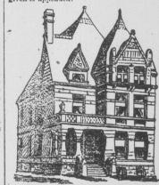
Brick or stone foundation, cut stone trimmings, slate roof; principal apartments finshed with hard wood, oil finish, inside blinds. etc. Height of stories—first, 10 feet 6 inches second, 10 feet. Cellar, 6 feet 6 inches in the
