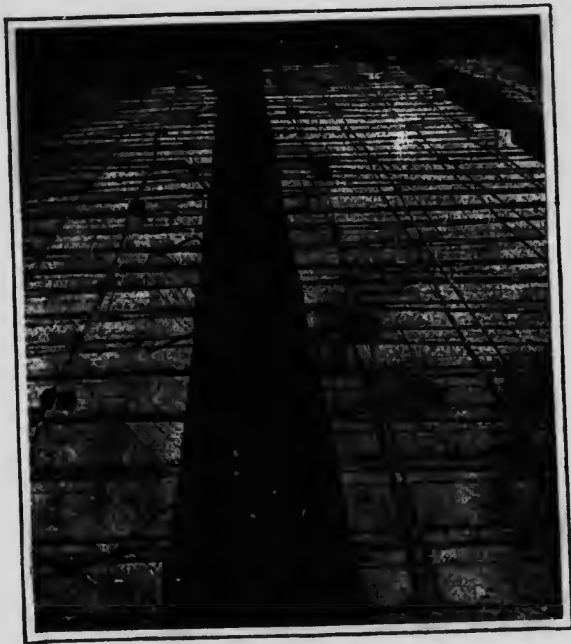
Fig. 8.—Wood Centering and Ransome Steel Bars for 50-foot Floor Span.
