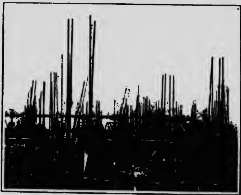
Fig. 7.—Ransome System of Erecting Columns.
