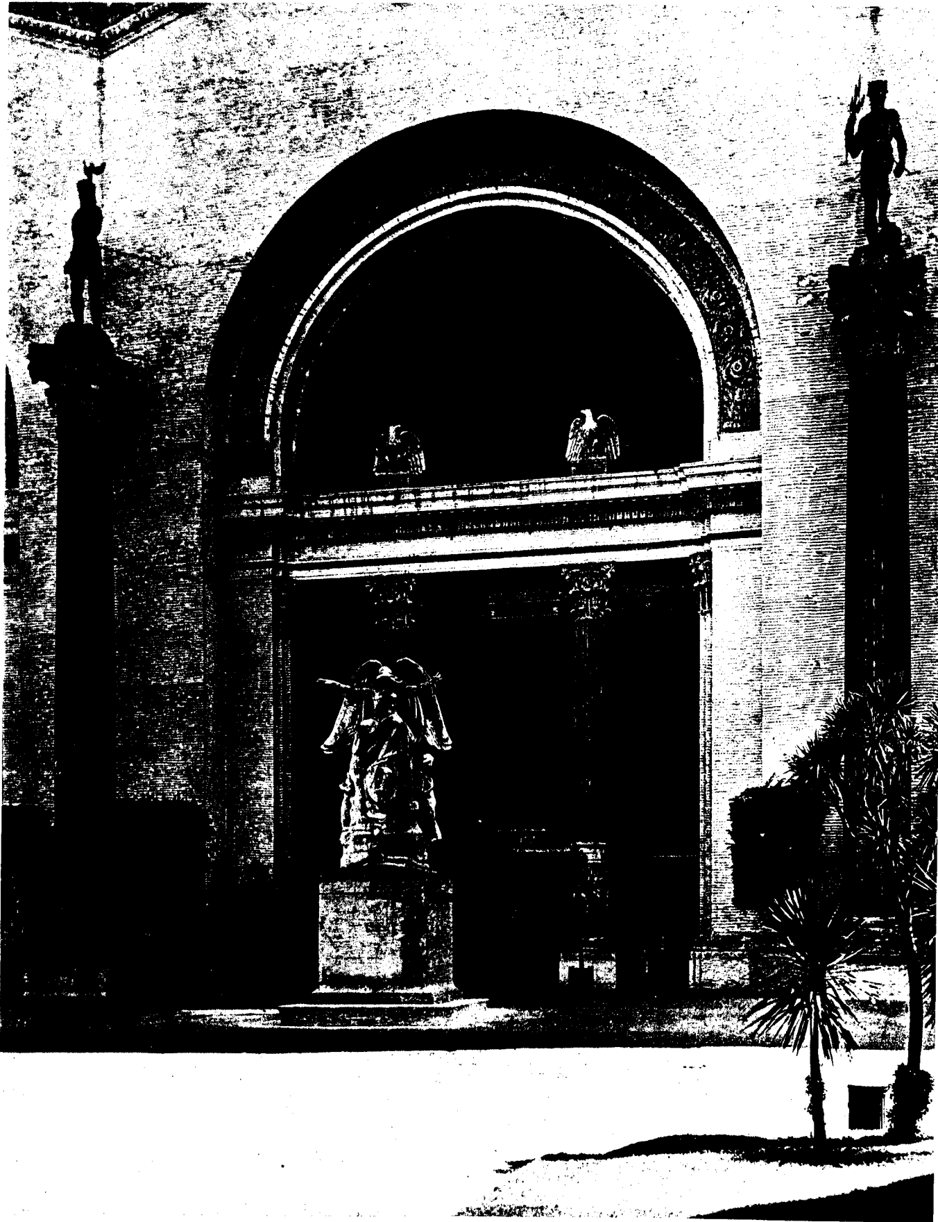
MAIN PORTAL OF THE MACHINERY HALL AT THE PANAMA-PACIFIC INTERNATIONAL EXPOSITION, SAN FRANCISCO, CALIFORNIA.
