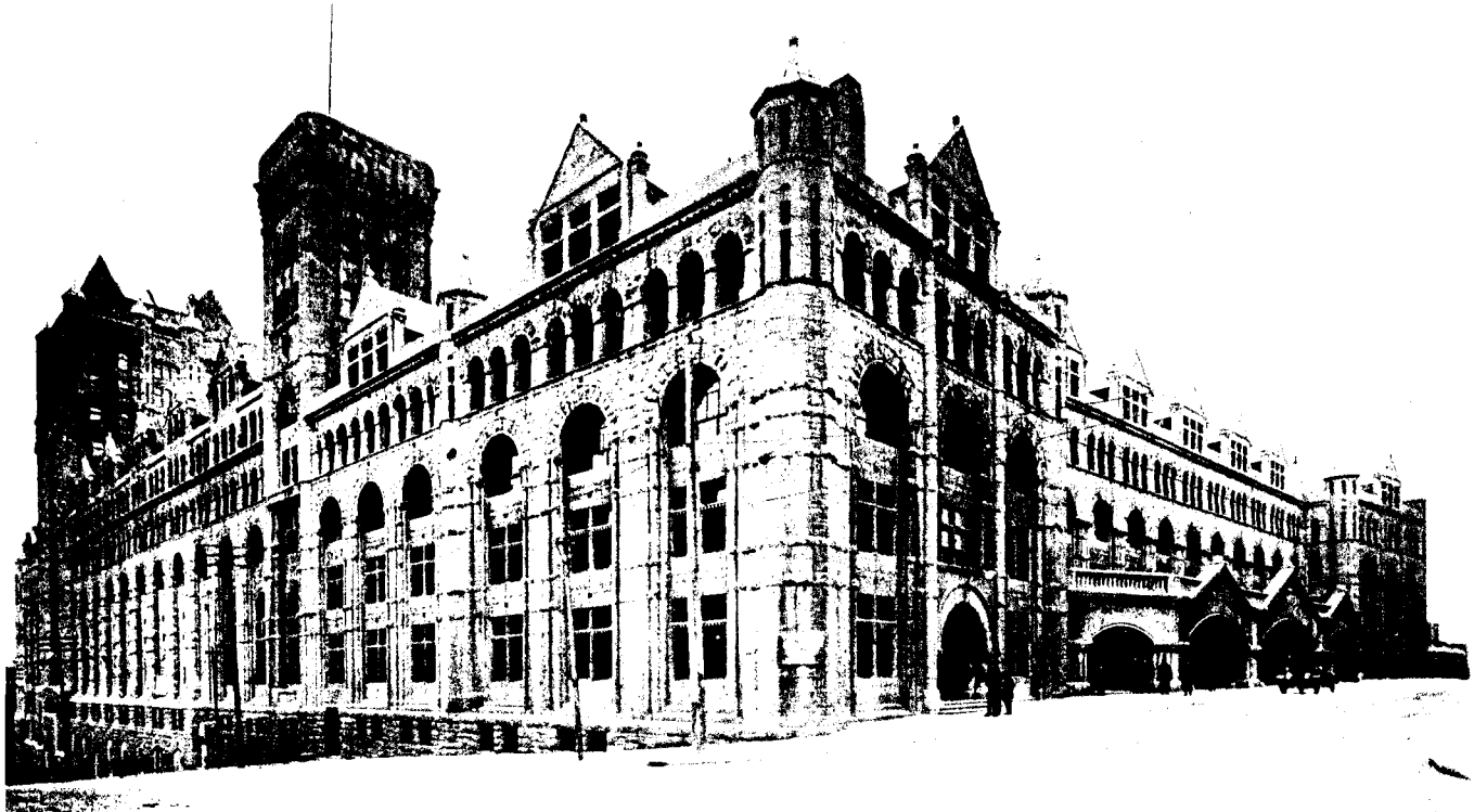
The new C.P.R. Windsor Street Terminal Station, Montreal, Que.
