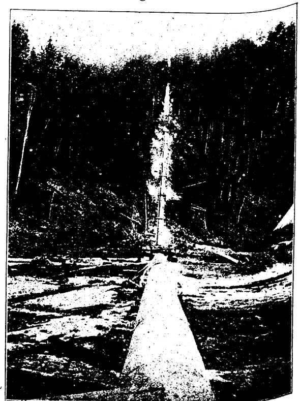
Steel Pipe Line Conveying Water to Monitors.
