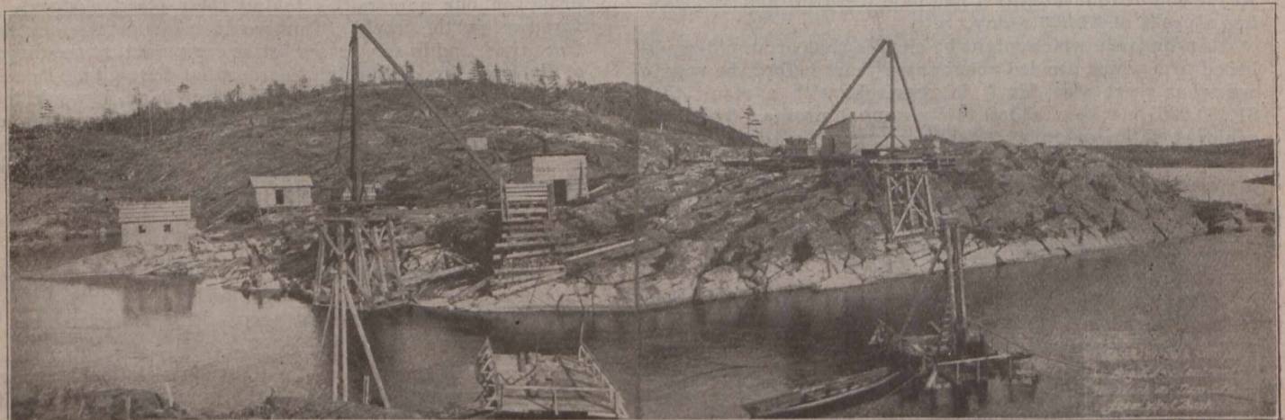
WORK AT DAM SITE—VIEW FROM WEST BANK
