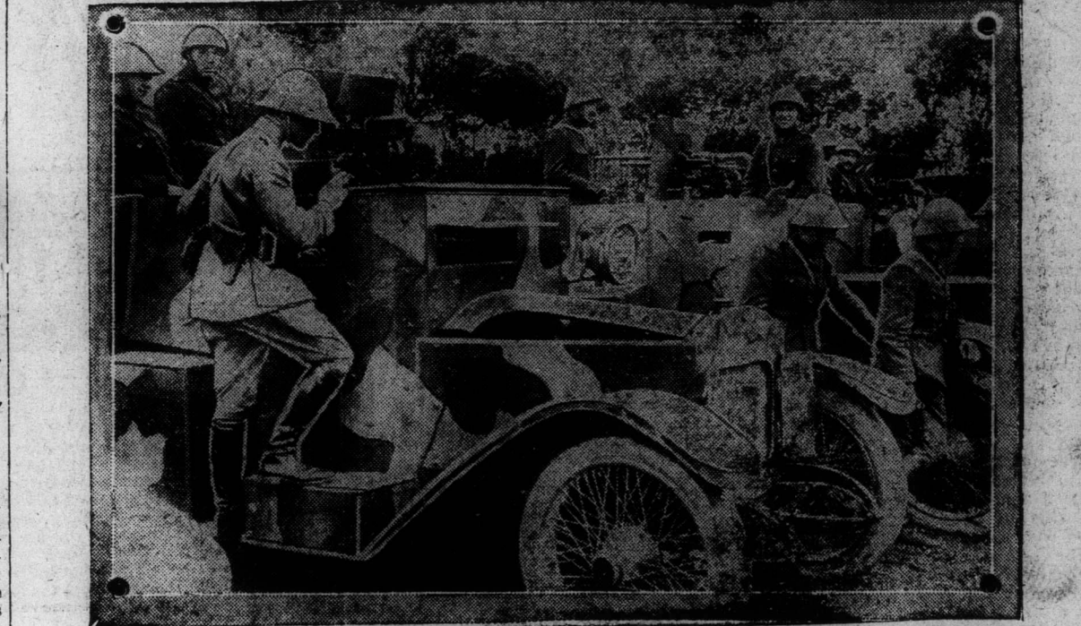
ONE OF THE NEW ARMORED MOTOR CARS MADE FOR THE BELGIAN ARMY. The picture shows one of the new armored motor cars transporting field artillery, and taking the place of the dog-drawn mitrailleuse used early in the war.
