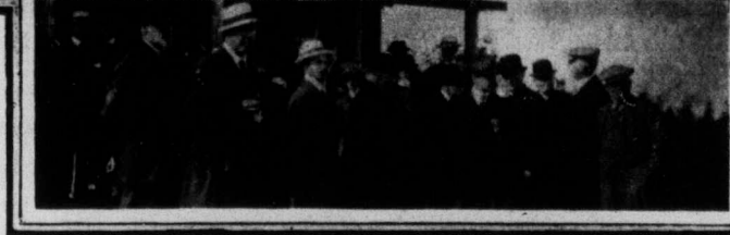
Convention delegates viewing car ferry construction work at Charlton.
