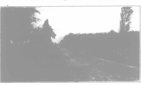
A clay road kept in excellent condition—during the summer of 1907, by John Young, Esq., Reeve of Caistor Township. A clay road can be kept at its best during the summer by using a split-log drag, but in the spring and fall, mud is inevitable. The roadside has also been neatly levelled.
