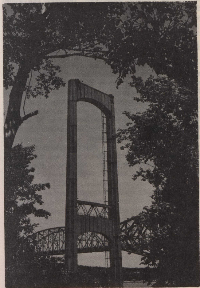
The two towers resting on the river piers rise to a height of 402 feet.
