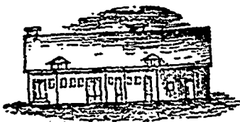
No. 5.—View of the Shops.
