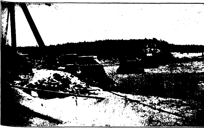
FIGURE 1.—SHUBENACADIE RIVER BRIDGE.
