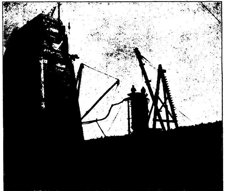
FIGURE 2.—PIER 1, SHUBENACADIE RIVER BRIDGE.
