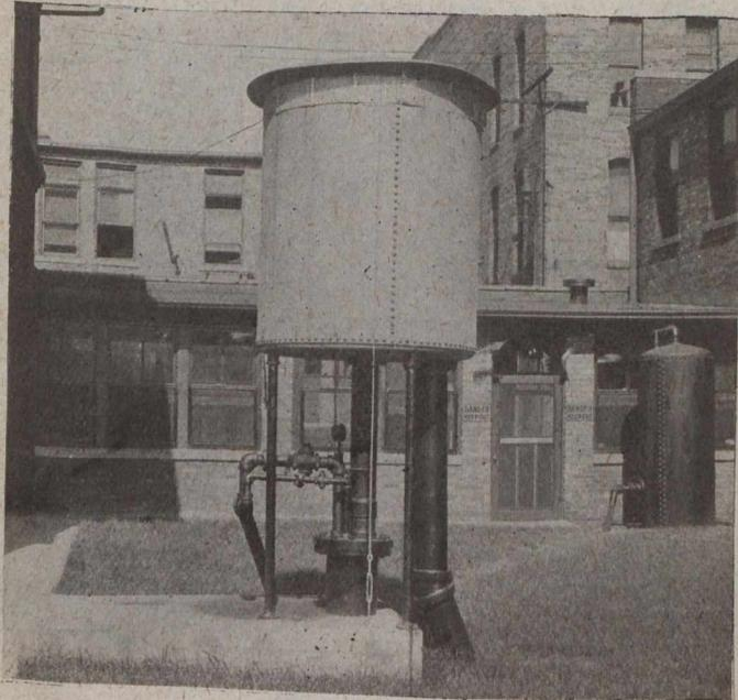
WELL-HEAD AND SEPARATING TANK AT GALESBURG, ILL.—AIR RECEIVER AT THE RIGHT
