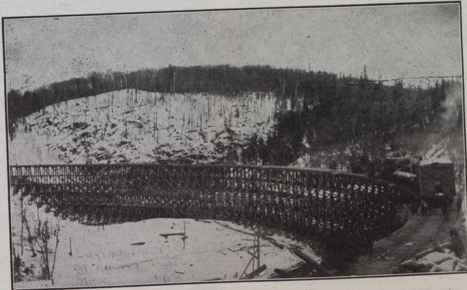
Laying Track on Algoma Trestle.
