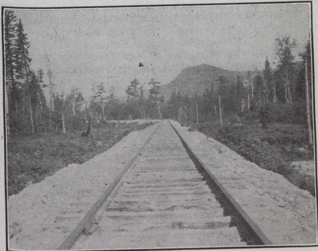
View of Roadbed at Mileage 87, S. C. & H. B. Ry.
