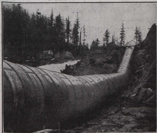
Fig. 5.—A Section of 12-ft. Pipe Line Manufactured by Ashmore, Benson and Pease for the Ocean Falls Power Company, British Columbia.
