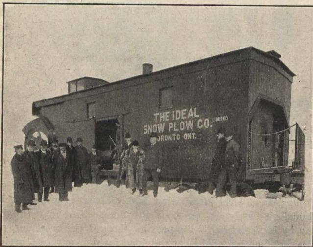
View Showing Location of Boiler.
