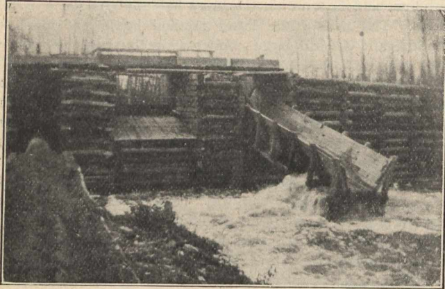
Dam Showing Timber Slide and Spill-Way.
