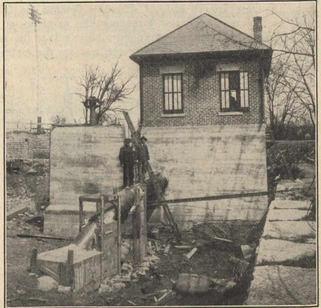
Lehman Street Pumping Plant.
